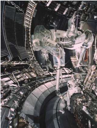
The present JET divertor MK II was installed using for the first time full remote techniques in a fusion device. Further modifications of the MK II divertor could be done with this technique as well.
