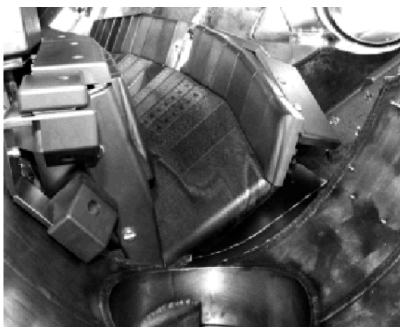
Lower Divertor Module of Wendelstein 7-AS
